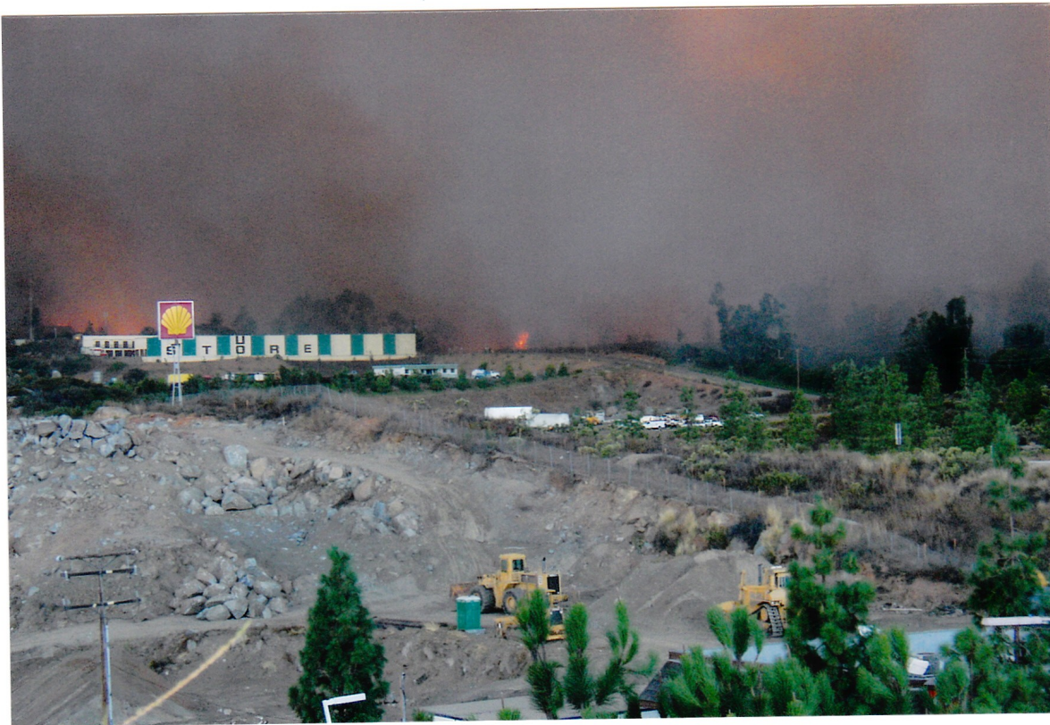
Looking toward U-Store Building
