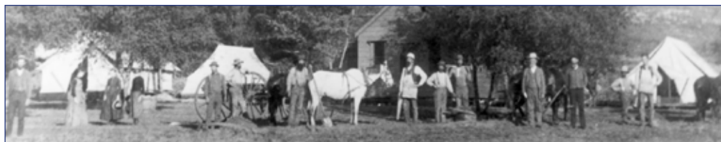
Local work crew building Arnold’s residence.
