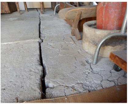
Priority 3: The concrete floor in the carriage house is severely cracked and uneven. This tripping hazard makes it unusable as an exhibit area. Funds are requested to remove the existing floor and install a new concrete floor.
